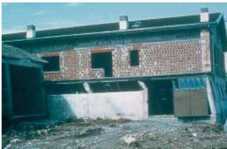
17/1 In this case, inserting parapet walls into a frame led to a short column phenomenon. Owing to the good confinement of the transverse reinforcement, no actual shear failure occurred, but an equally dangerous sway mechanism developed (Friaul, Italy 1976).
