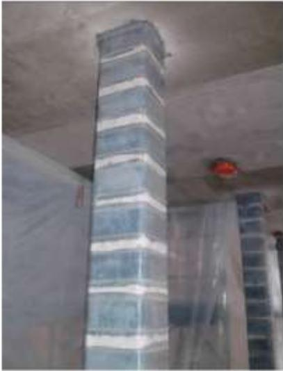
carbon fibres wrapping to increase the shear strength in a column
