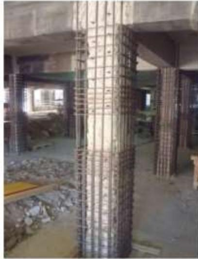
concrete casting to increase shear and flexural strength
