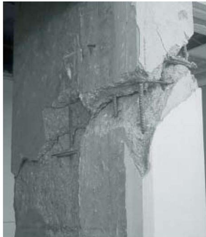
17/3 Better transverse reinforcement in the column (small spaced hoops and ties) would probably have prevented the shear failure. However, the source of the problem lies in the partial infilling of the frame that caused the short column phenomenon (Izmit, Turkey 1999).
