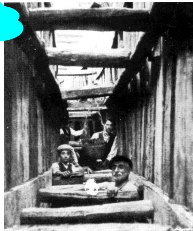
Figura 40. Timbering in Deep Trench
