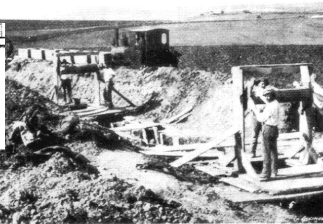
Figura 39. Excavation of Trench on Foggia Branch
