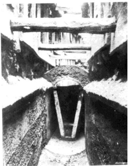
Figura 38. Construction of Canal in Earth
