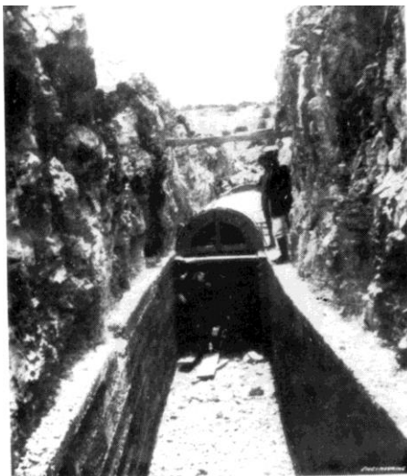
Figura 37. Construction of Canal in Rocky Ground
