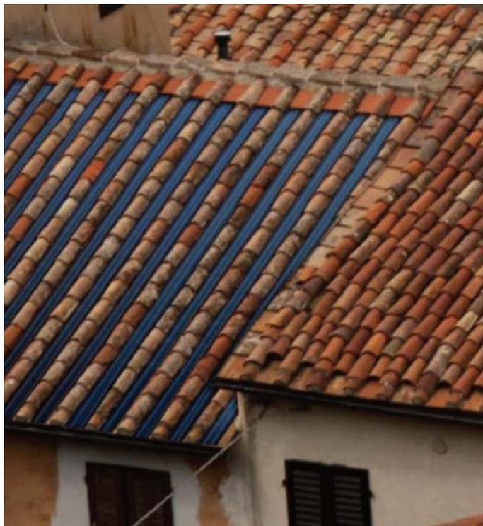
Solution by vertical installation of PV panels on Mediterranean roofs (System provider: Hemera)
