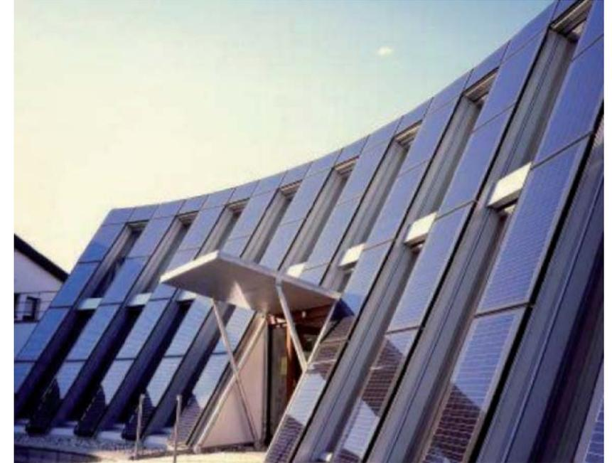
Juwi Head Office, Bolanden (Germany): ideal façade inclination with large-scale PV modules to harvest a maximum of solar energy (Surface: 70 m<sup>2</sup>, Energy output: 7.2 kWp, System provider: Schüco International KG, 2004)
