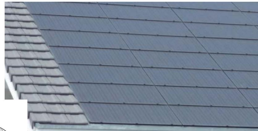
**Energy Roof is an integrated solar PV system that uses an innovative framing structure to convert conventional roofs into electricity generators.**
