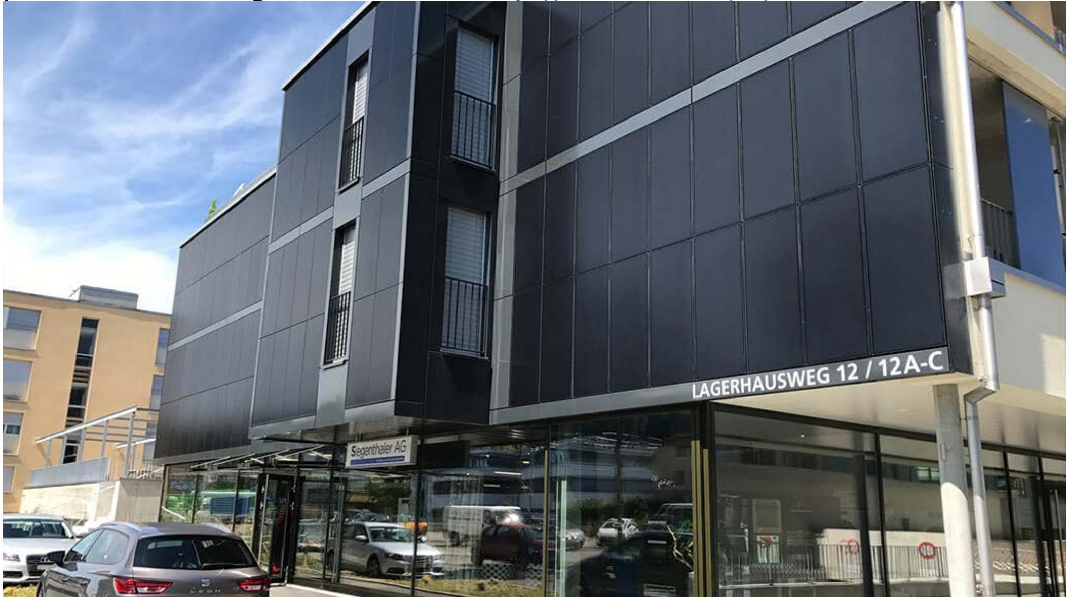
Torgau (Germany) / Lyss (Switzerland), August 2nd, 2017 – AVANCIS, one of the leading manufacturers of premium CIGS PV modules, demonstrates the power of its thin-film modules in the BIPV area. The solar façade of the new building at Senn Areal in Bern, a residential and commercial building, now produces its own electricity. The façade generates a total solar power of 12 MWh per year current on 135 sm by 130 PowerMax® SKALA PV modules.
