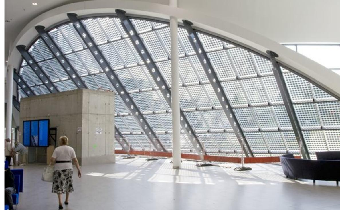
It is a solution that is enabling a Belgian hospital, O.L.V.-Ziekenhuis in Aalst, to generate substantial amounts of solar energy for their own use. Every square meter produces 100 watts of power and the total net surface area of the photovoltaic cells is 500 square meters
