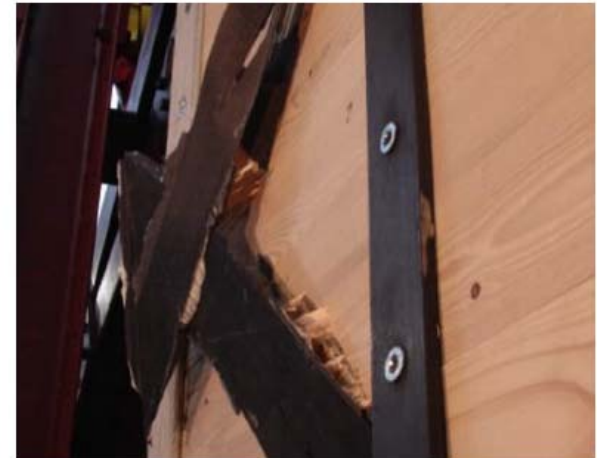
Fig. 18. Failure mechanism of specimen F4 with CFRP strips detachment.
