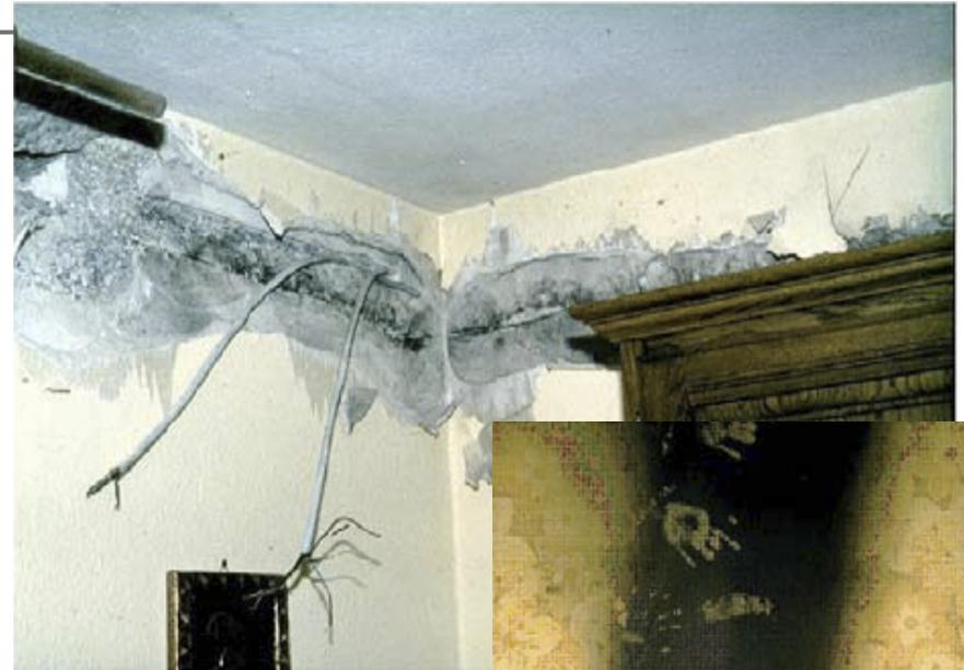
**Punctures to concealed cables due to lightning strike**
