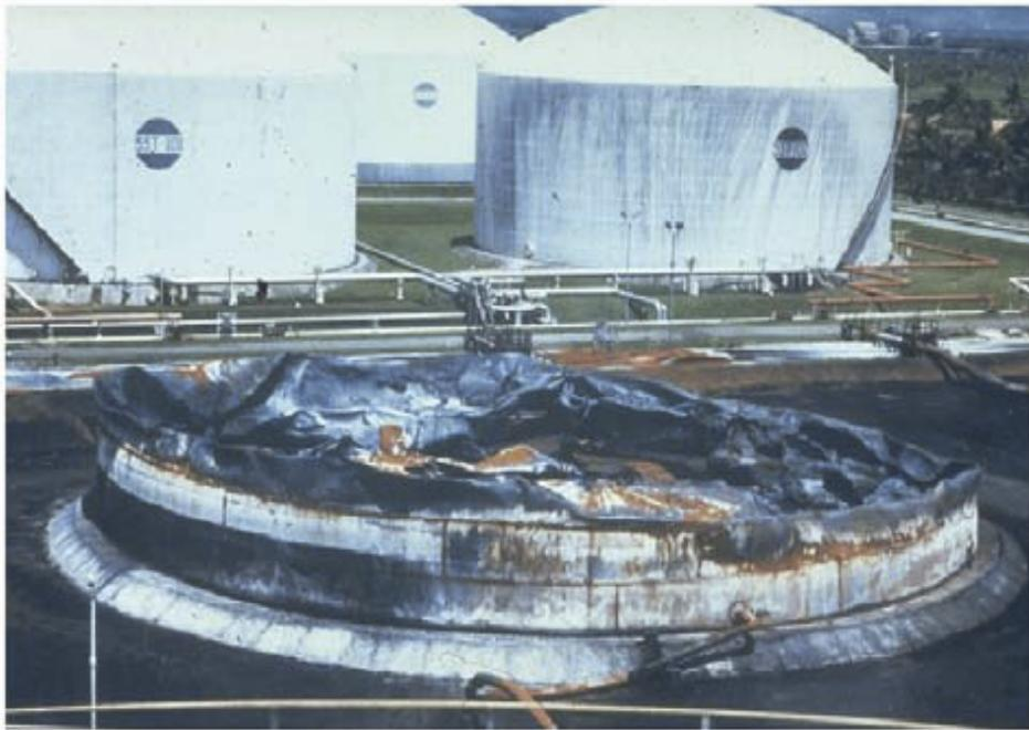
**Tank explosion caused by lightning Cilacap / Java 1995**
