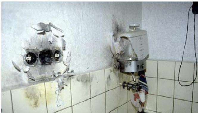
**Boiler damaged by lightning strike**
