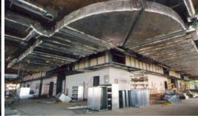
Construction Progress Monitoring
