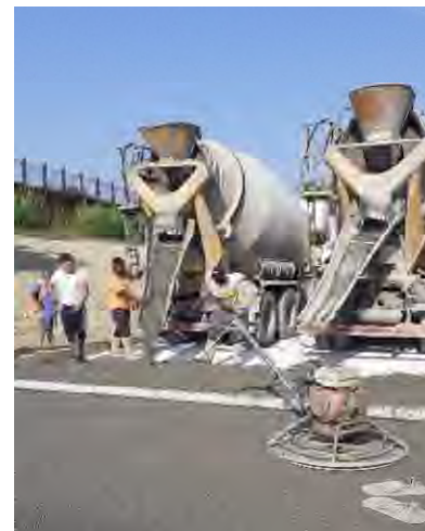
Posa in opera
