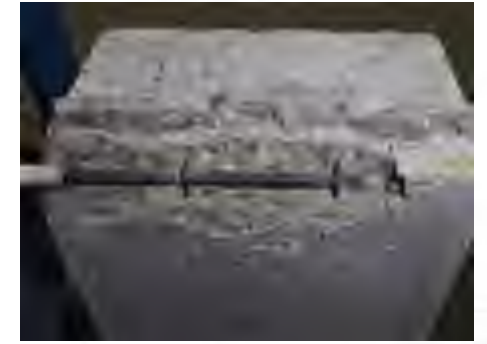
Side-face splitting failure
