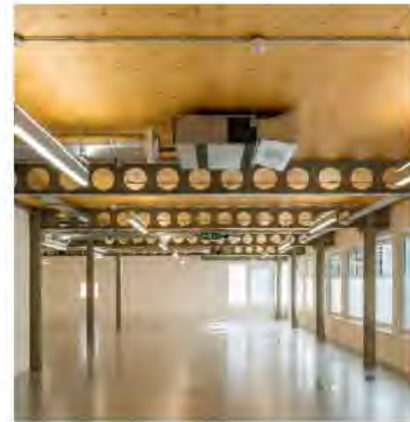
SYSTEM 3: TIMBER AND STEEL
