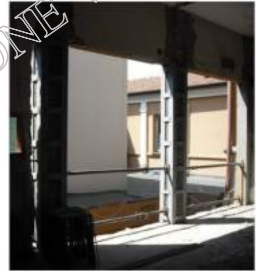
steel encasing for the same purpose
