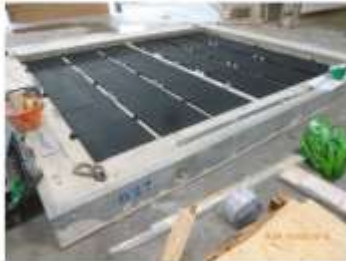
Pose des panneaux / Pose of panels Arco FIBER
