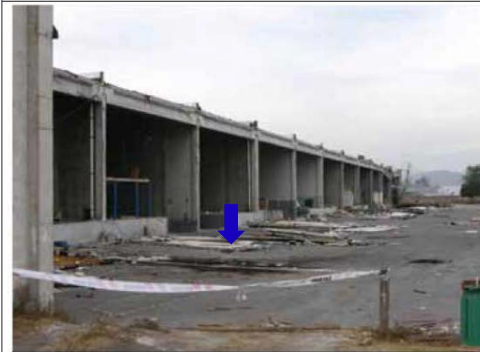
**Figure 13.** Rear elevation of the same office and warehouse building showing fallen exterior walls and exposed transverse walls and end columns.
