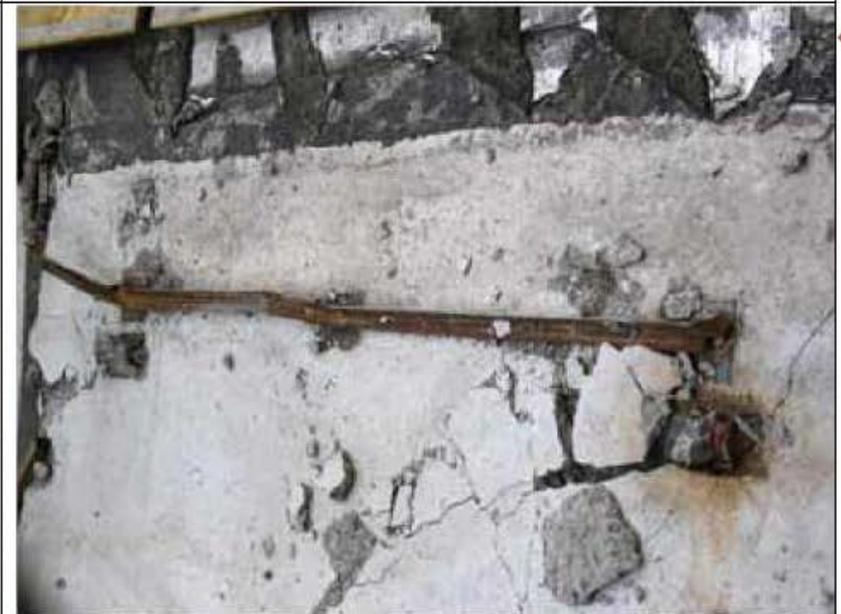
**Figure 15.** Bent and broken connection angle that failed to hold walls to edge beam at roof.
