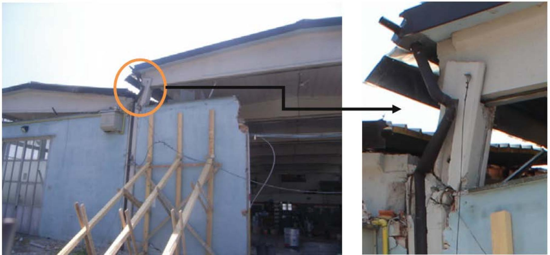
**Fig. 10** Loss of the left girder seating due to the interaction with masonry panels (short columns/shear failure)
